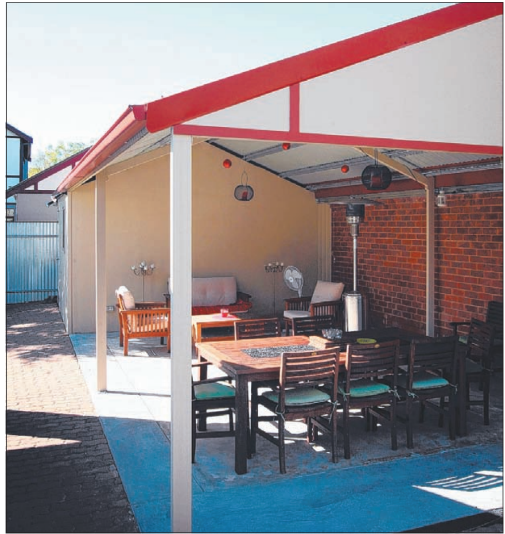
OPEN PLAN: Ray Webster, inset left, combines outdoor living, above, with traditional storage, pictured on the cover, in his shed.
